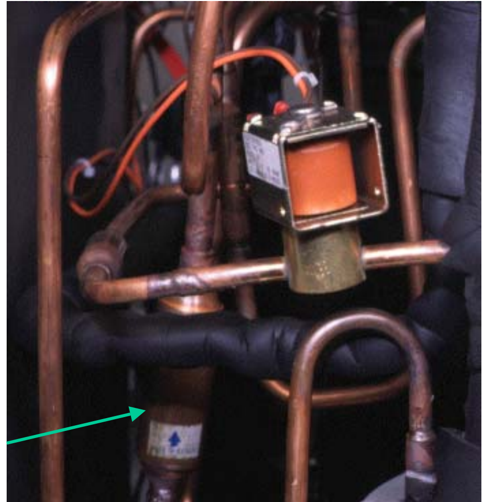
Discharge Line Check Valve
